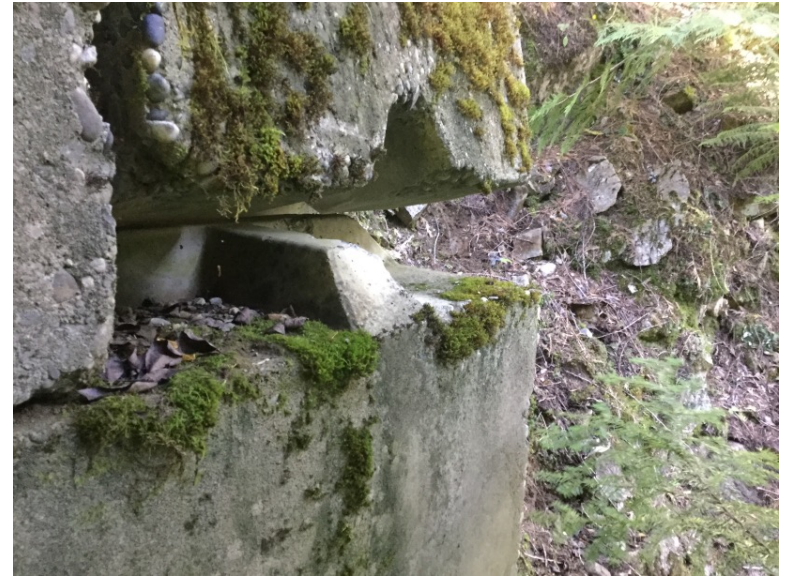
Upstream right bank bearing block condition
