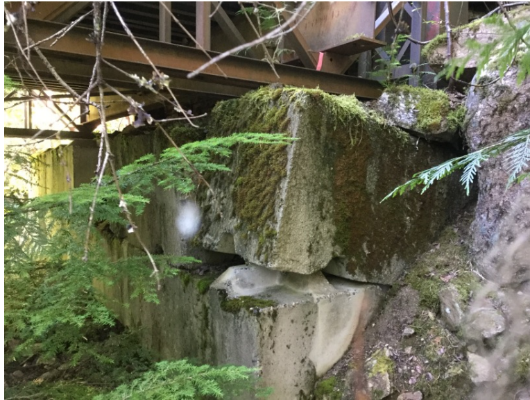
Upstream right bank bearing block condition
