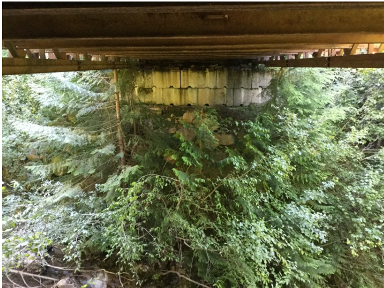
Left Bank Abutment when facing downstream
