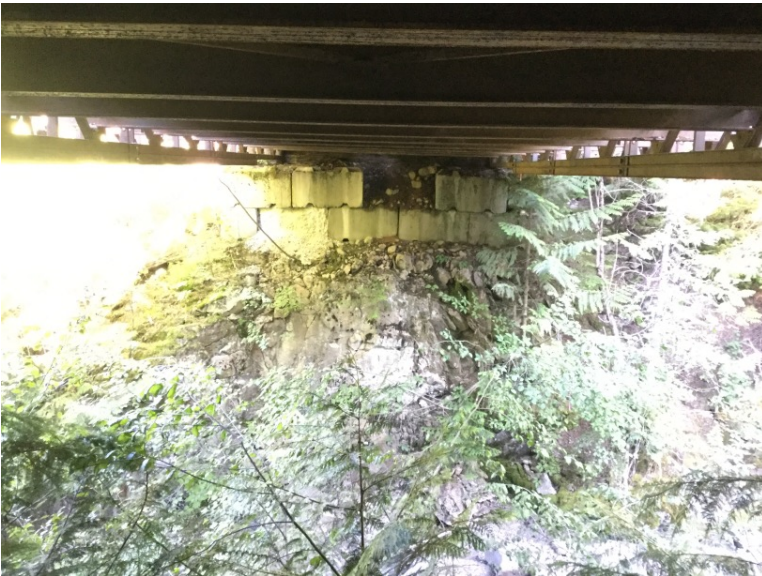
Right Bank Abutment when facing downstream
