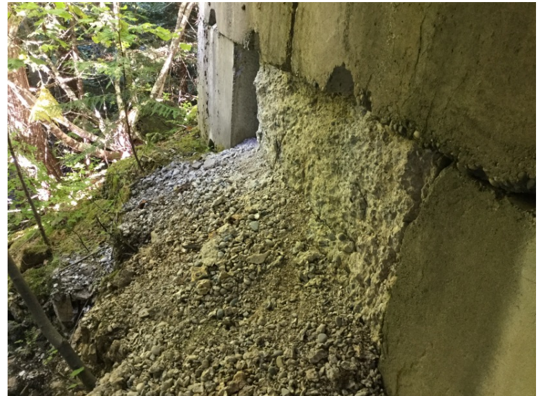
Lock block condition at downstream right bank
